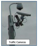
The CCTVs monitor traffic conditions, provide monitoring, and/or verification of traffic congestion and incidents, and verification of traveler information messages. The MVDS monitors, collects, and processes traffic data, including volume, speed, and lane occupancy. Traffic data gathered from this detection
