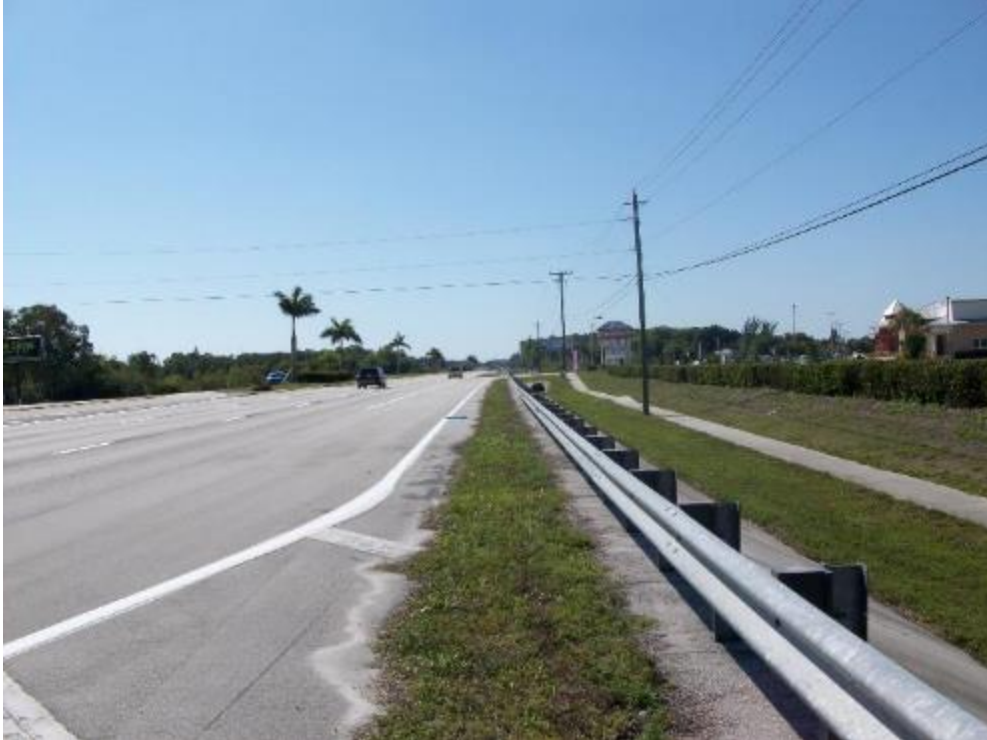
Photo 8: Keyhole at Harbour Plaza will require 54" pipe to be extended and ditch to be filled.
