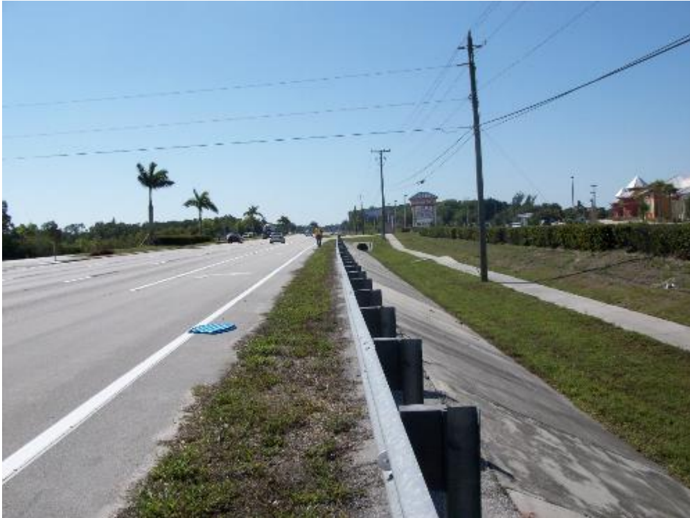
Photo 4: Slope pavement and guardrail to be removed for keyhole at right-turn to Harbour Plaza
