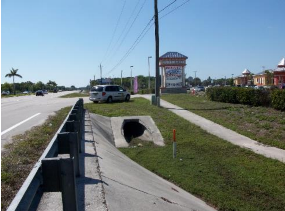
Photo 6: Keyhole at Harbour Plaza will require extension of pipe.
