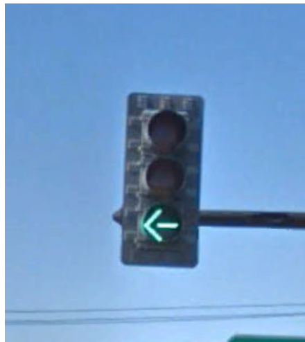
Backplate Present No retroreflective sheeting
