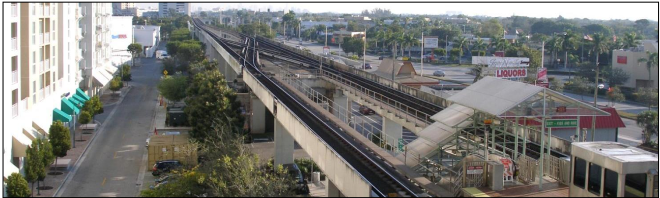
Metrorail, looking northeast from Dadeland. South Dixie Highway (US 1) is to the far right.
