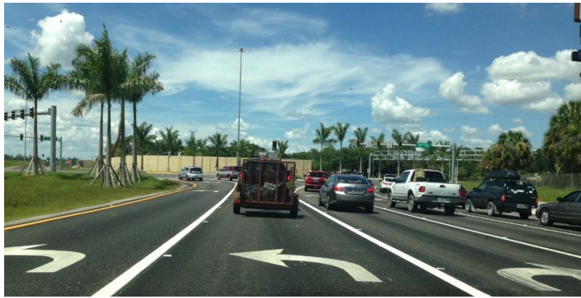
SR 80 Interchange - Northbound exit ramp from I-75 to SR 80
