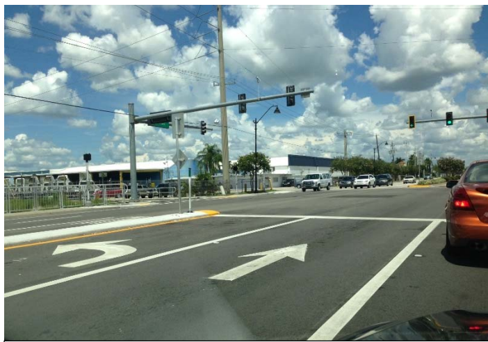
New separator and eastbound left turn lane on MLK @ Veronica Shoemaker
